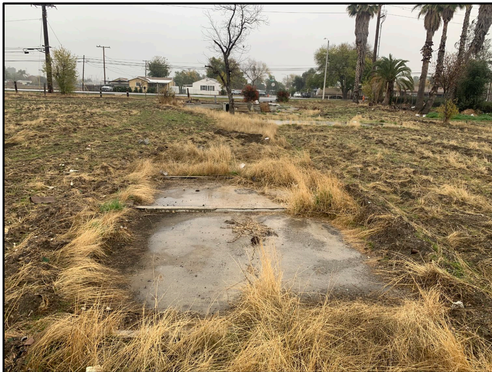
Plate 3.2–19: Overview of the concrete pads, facing east. The western-most concrete pad is in the foreground and the central concrete pad is in the background, in front of the foundation.
